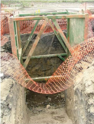
Typical Ground Conditions – Heavy Clay
